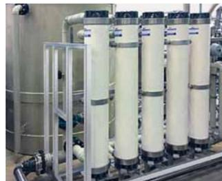
Removal of colloids and bacteria by means of ultrafiltration
